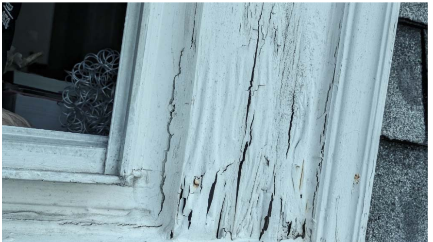
IMG. 13-810 Failing Caulk (Typ. for All Windows); Window and Storm Door in Need of Paint (Typ. for Most Original Wood Windows) at Unit 13. Repaired since by Owner
