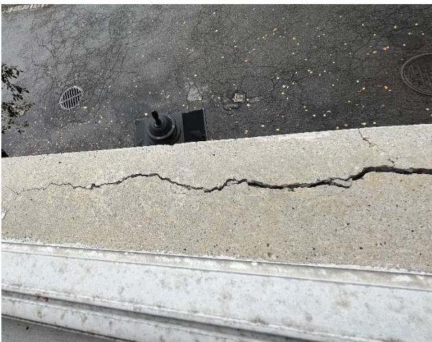
IMG. 1-710 Deteriorated Brick and Mortar Caused by Backsplash Unit 1
