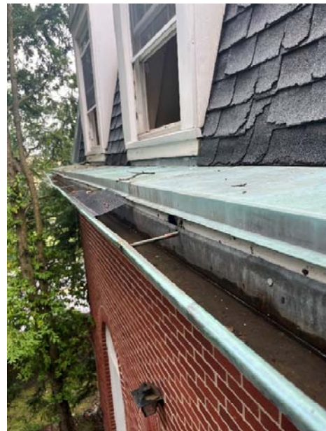
IMG. 16-210 Expired Roof Membrane & Mansard Shingles; Improper Flashing/Dormer Top Repairs Units 16/17/18 IMG. 21-310 Gutter Detached/Damaged/Clogged Unit 21
