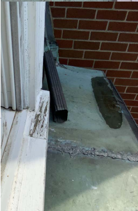
IMG. 14-310 Badly Maintained Cornice Flashing Unit 14 Back IMG. 11-310 Poorly Repaired & Dented (Puddling) Cornice Flashing; Incorrect Leader Installation Unit 11 Front
