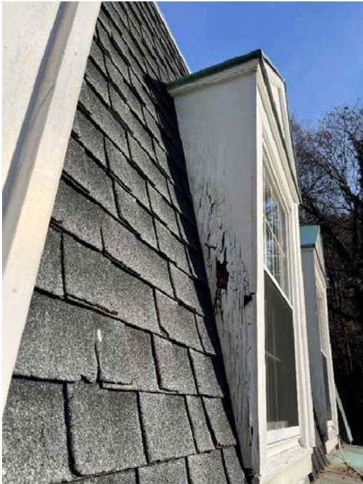
IMG. 13-410 Failing Mansard Shingles Unit 13 Back
