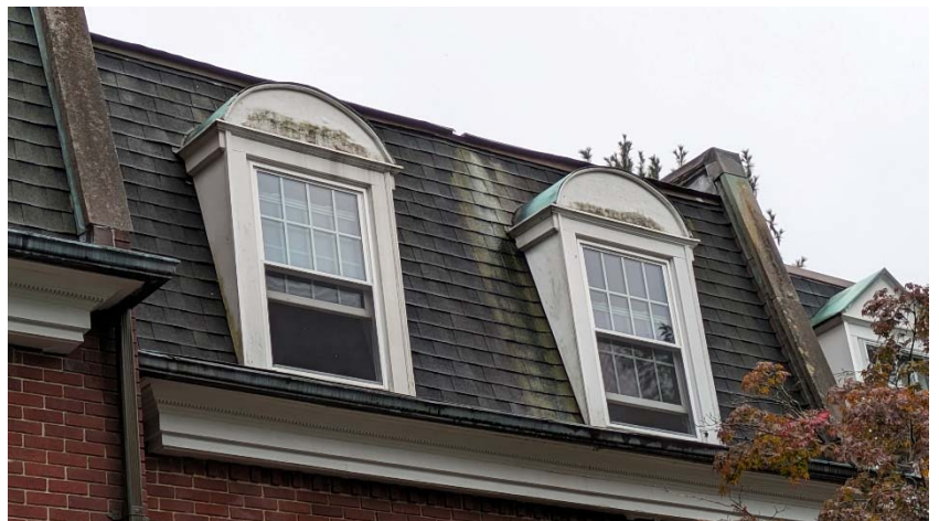
IMG. 19-400 Expired Mansard Shingles; Spilling & Incorrectly Installed Leaders Unit 19 Front
